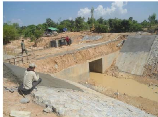
Spillway constructed to keep water in the canal and to bring more water to the lake reservoir in the target area of CCBAP.
