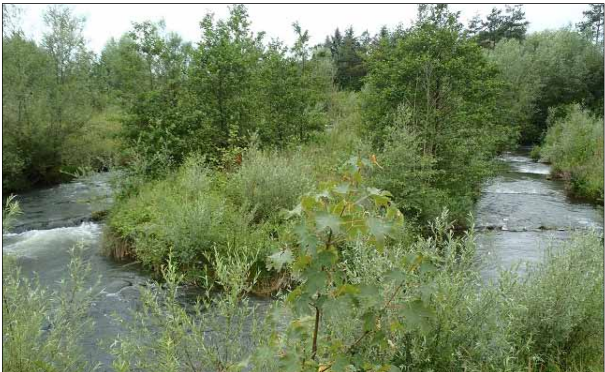
Figure 26: Nature-like fish pass at Kemmelbach Hydropower Plant on the River Ybbs in Austria (© Mielach)
