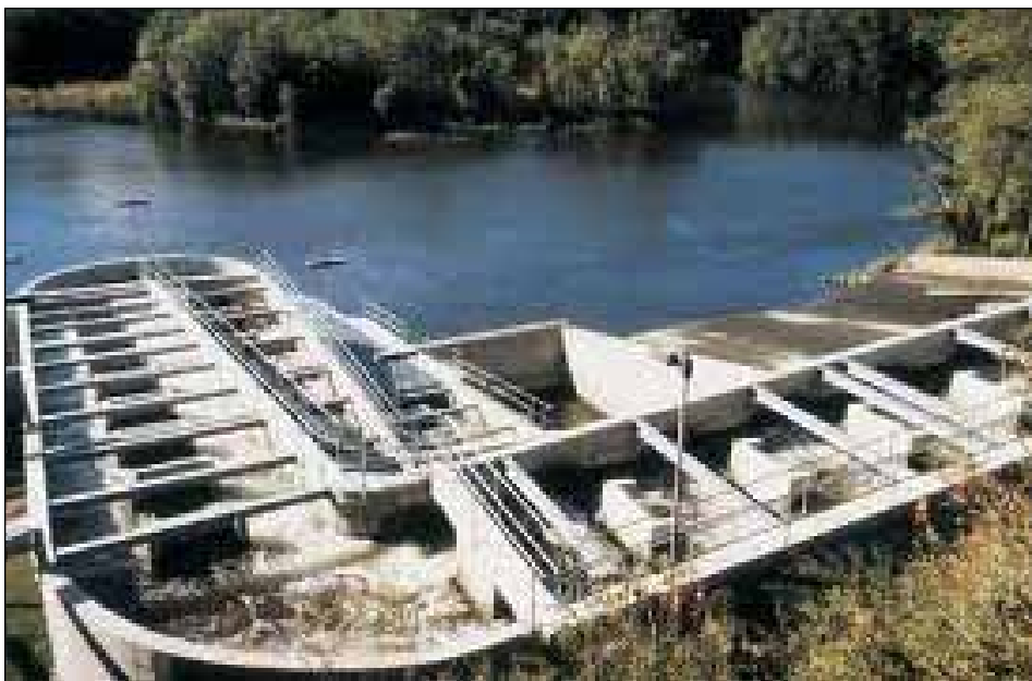
Figure 36: Yangtang Fishway at the Mishui River (www.fao.org)
