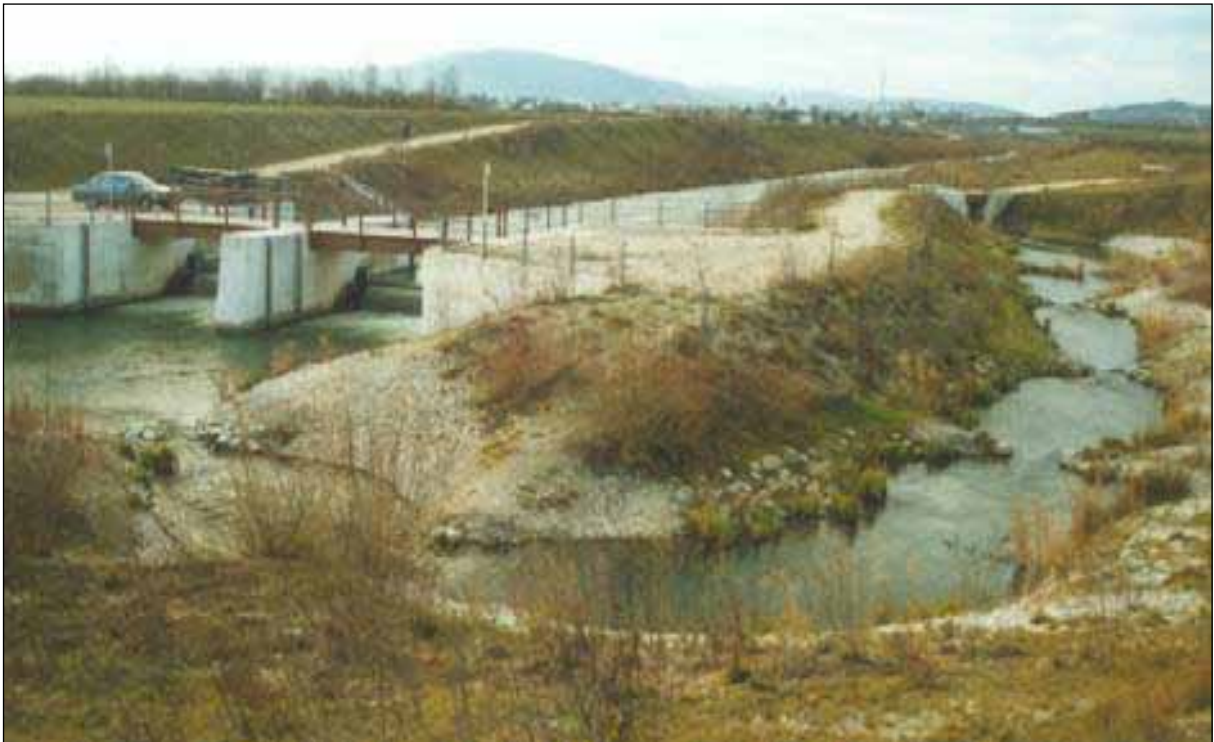
Figure 29: Nature-like fish pass at Marchfeldkanal, side channel of the Danube River, Austria
