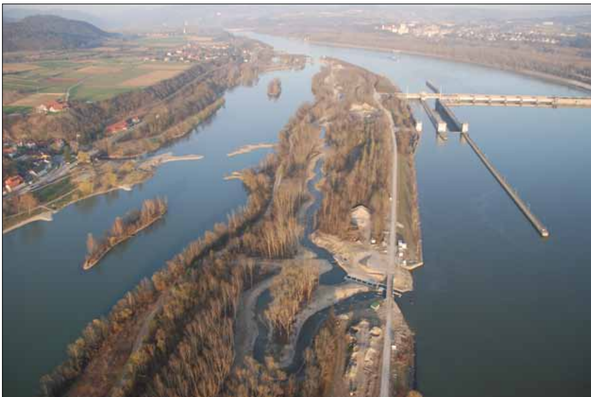
Figure 30: Melk Fish Pass on the Danube River (© Verbund Austria AG)
