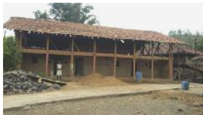
Figure 5. Farmer building his house with Tectona grandis (teak) extracted from adjacent, remnant forest (probably illicitly). (Photo: James Brockington)
