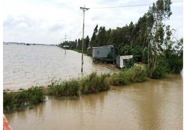
Figure 9 D. Flood discharge after summer-autumn rice crop in Tan My, Thanh Binh, Dong Thap (16/08/2018). It can be clearly seen that the embankment was very low.
